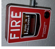
Typical Pull Station
